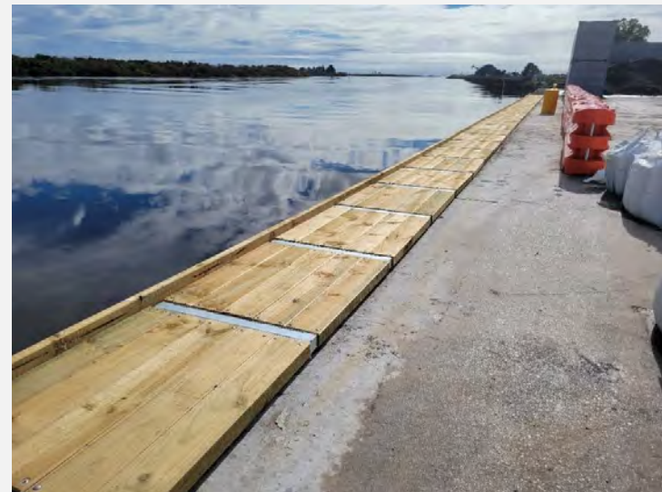
New strengthened wharf edge to support on-going use
