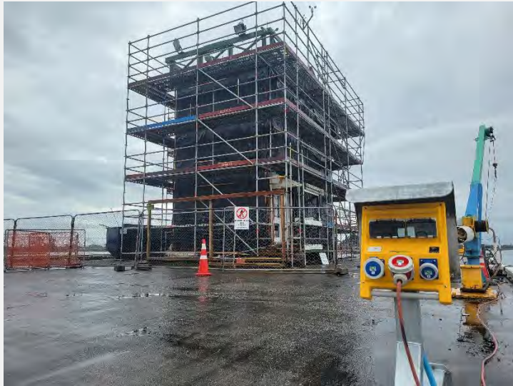
Harbourmaster office (before/during)
