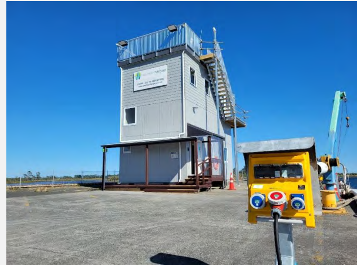
Harbourmaster office (after)
