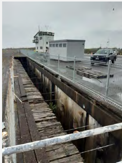
New safety fencing to isolate hazardous areas of the Port
