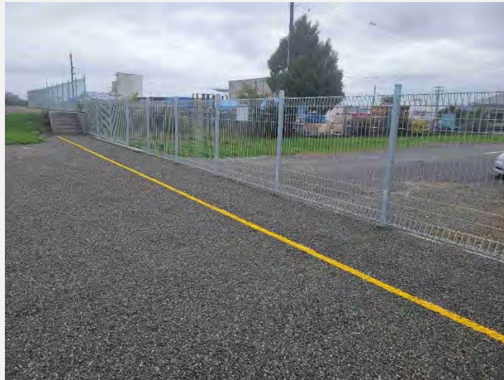
Example of extensive new perimeter fencing for security and control
