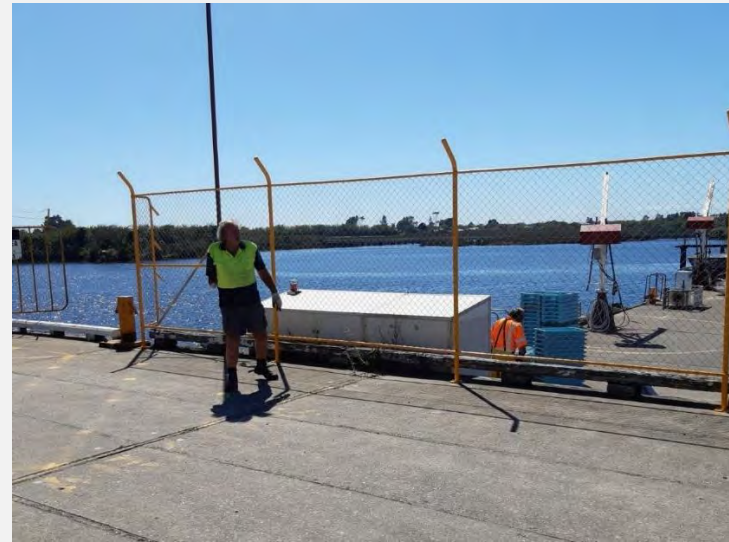
New fall protection fencing separating wharf entities
