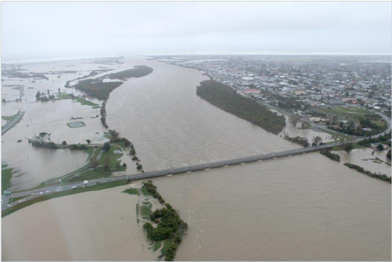
Figure 8 - Flood waters at the Buller Bridge, July 2021
