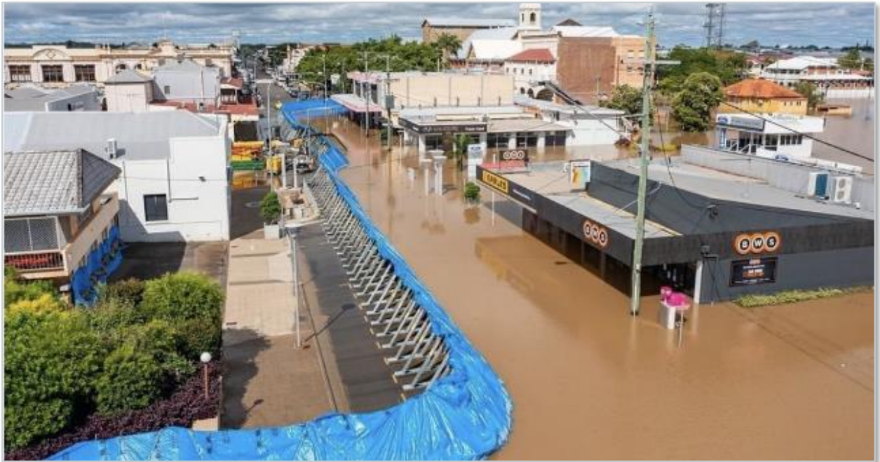
Figure 29 - Inflatable temporary flood barrier
