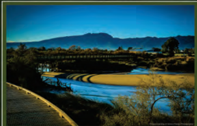
Boardwalks Westport Harbour
