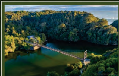
Nile River Bridge, Charleston Kawatiri Coastal Trail
