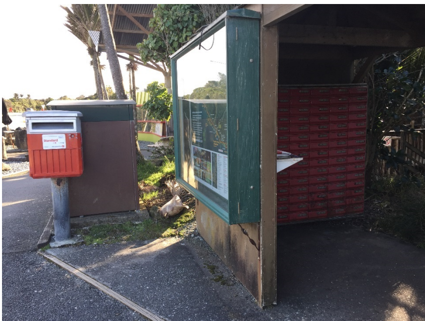
Figure 3-9: Existing community mail facilities at Dolomite Point
