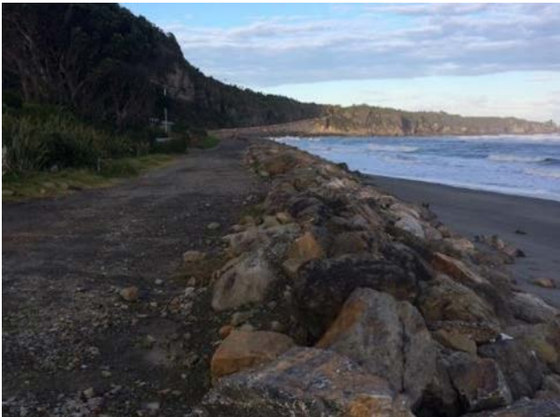
Figure 3-16: Seawall protection at Punakaiki
