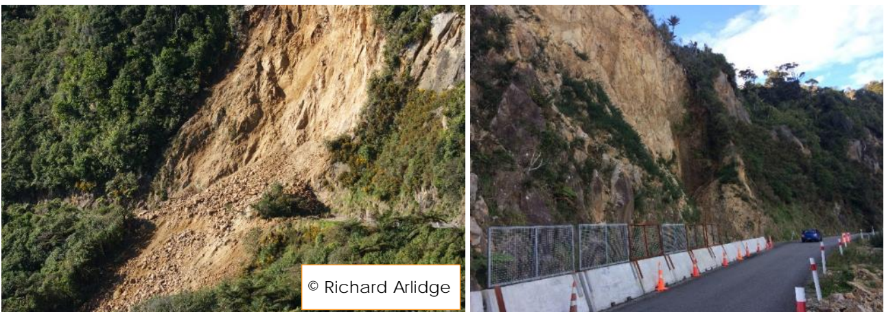
Figure 3-4: The scale of the landslip that closed SH6 in September 2016
