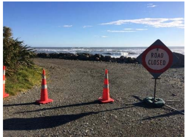
Figure 3-17: Dickinson Avenue is now closed as a result of coastal funding
