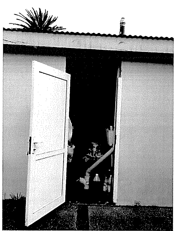
Guttering required on building
